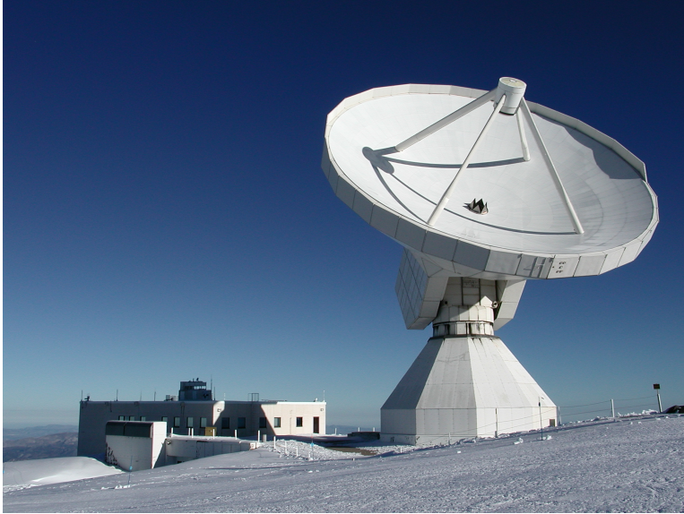
Figure 2.1: IRAM 30 m telescope - Located in Pico Veleta, Granada (Spain), it is a 30 m single dish parabolic antenna observing at 0.8, 1, 2, and 3 mm. Credit: IRAM.
